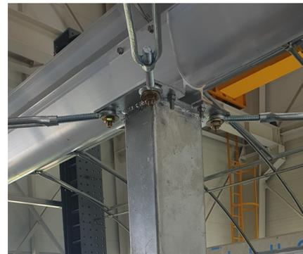
Fig. 1. Configuration of bracing member connection.
