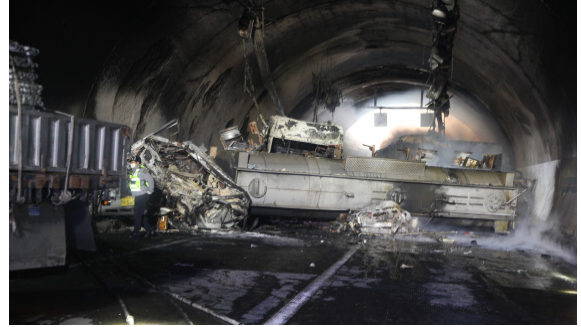
(b) Underground tunnel fire (Samae 2 tunnel, 2020)
