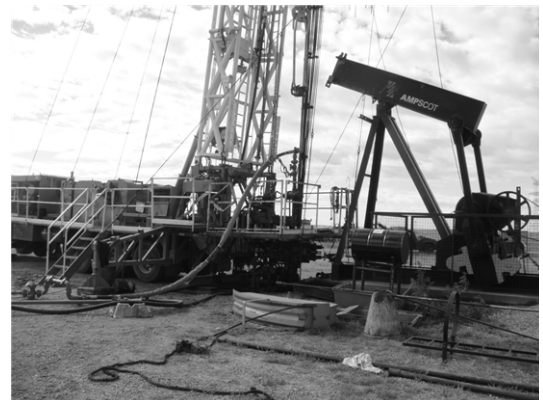
Fig. 7. Pump injection line.
