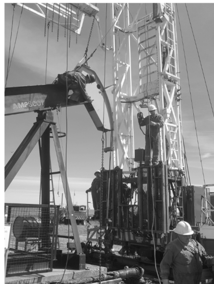
Fig. 3. Removal of sucker rod head using workover service rig.
