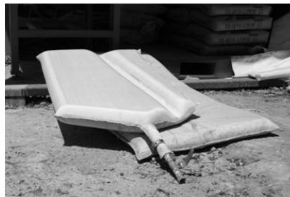
(b) Pressurization bag after grouting
