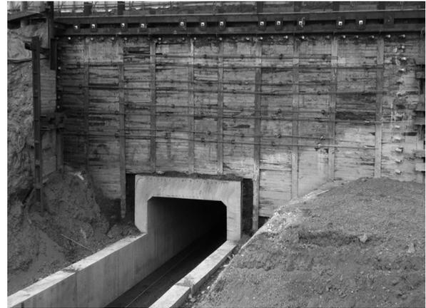
(b) concrete channel box in the excavated area
