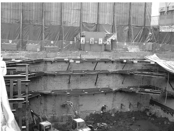
Photo 1. IPS earth retention system applied in soft clay
